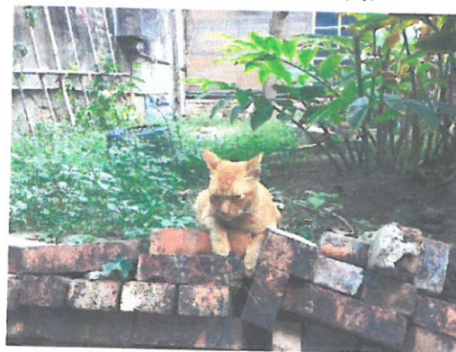
/舊磚塊的鋪設鬆動/
